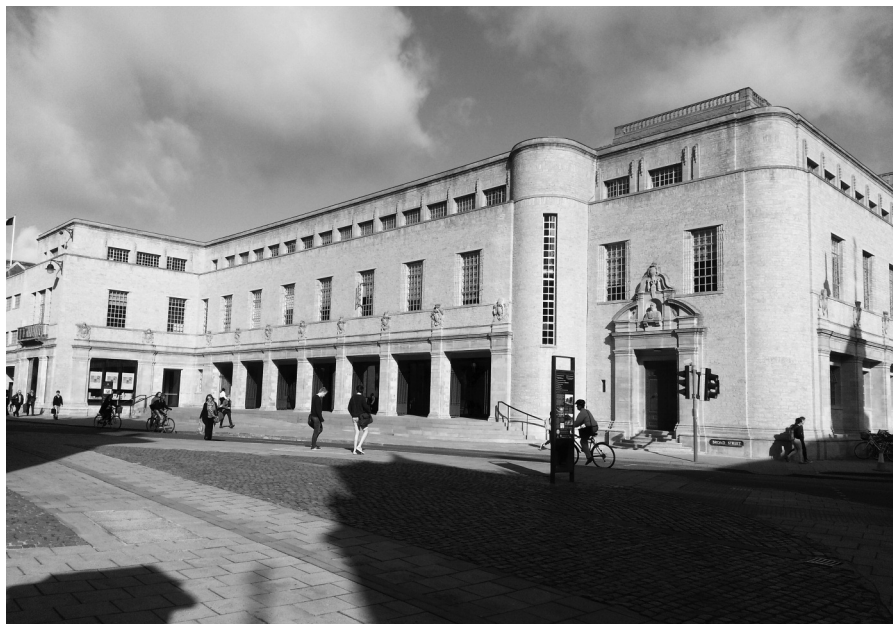
Fig. 1 Exterior from Broad Street
